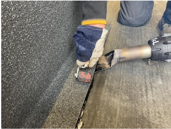
Fig. 14 Lassen overlap opstand met warme lucht
